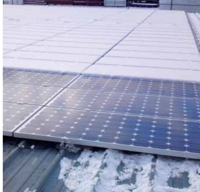
↑ Heavy snowfall complicated the installation
